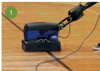
1 Clean floor with Bona DeepClean W using Bona PowerScrubber. Let it dry
