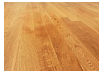
Floor is revived and fresh looking once again
