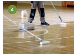
4 Apply Bona Sportive Finish using a roller
