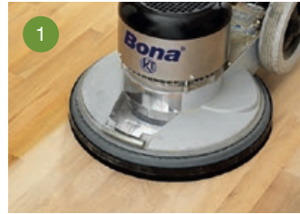
1 Sand the floor with Bona Flexisand or Bona Belt.
