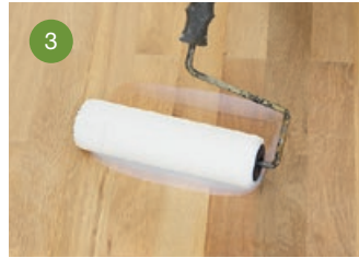
3 Use a Bona Roller and apply first layer of Bona Mega ONE.
