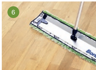
6 Remove sanding dust with a Bona dusting pad or a Bona DCS25.
