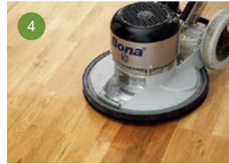
4 After only 1 hour, mid abrade with Bona FlexiSand.
