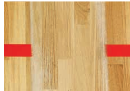
Bona 8700 effectively removes old finish / line marking
