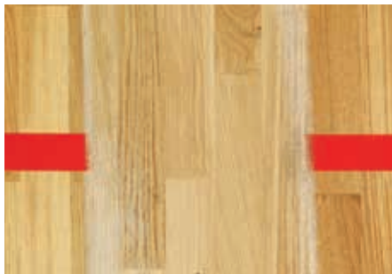
Bona 8300 effectively removes old finish / line marking
